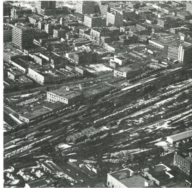
The proximity of the CP Rail yards to Regina's downtown business core is seen here. The release of this land will give Regina a unique opportunity to redevelop its downtown area.
