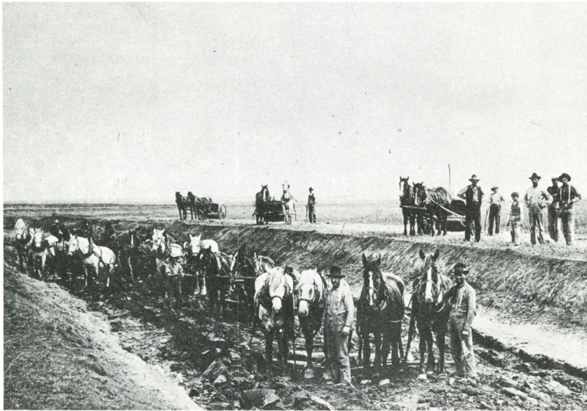
Railroad levelling through the wheat fields of the Canadian Prairies (circa 1905). Photo: Public Archives of Canada.
